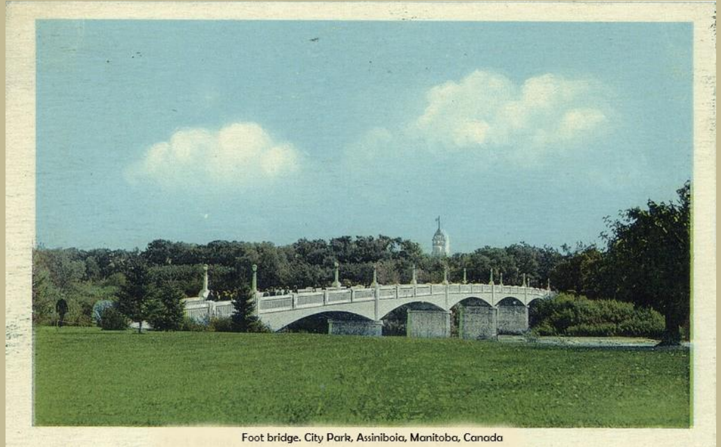
Foot bridge. City Park, Assiniboia, Manitoba, Canada
